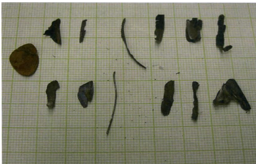
Figure 1 Foreign bodies in the pipes of the sprinkler system
